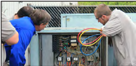
HVAC Training at Regional Occupation Center.
